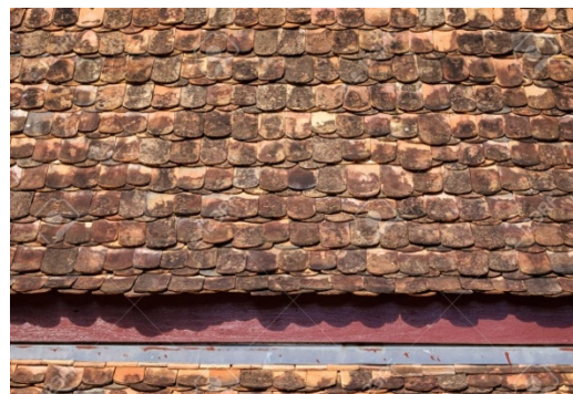
Gambar 7 : Susunan pemasangan atap genting Sumber : https://www.123rf.com/photo_ancient-roof-tile-thai-temple.html
